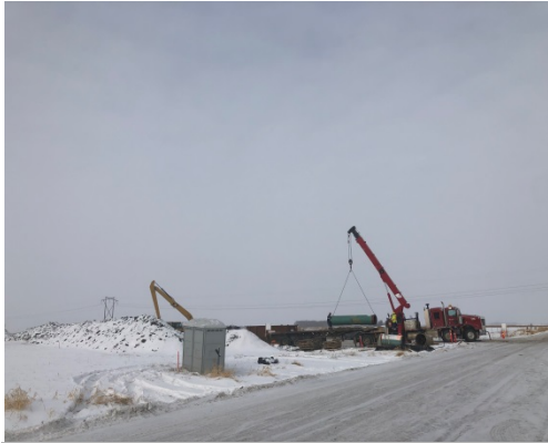
SF 22B, photo facing north west, boom semi truck loading up short pieces of pipe.
